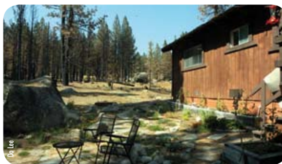
This property shows some options for defensible space such as rock pathways and low growing plants near the house.
